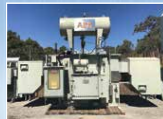
EL3327 15,000 KVA ABB Transformer: 33,000 to 11,000 Volts - Dyn11 - Complete with OLTC
