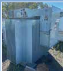
EL3388 2500 KVA ABB Transformer: 11,000 to 433 Volts – Dyn11
