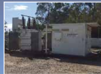
EL3298 6000 KVA Power Plant & Process Substation: 66,000 to 11,000 Volts - Dyn11- Complete with 66 KV Circuit Breaker
