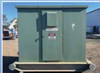
EL3407 500 KVA Ramsay Kiosk Transformer: 11,000 to 433 Volts – Dyn11 – Dry Type.
