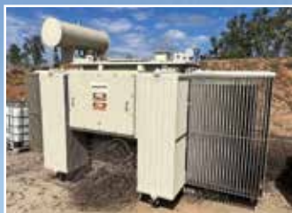
EL3406 5000 KVA QTC Transformer: 11,000 Volts to 6600 Volts – Ynd11
