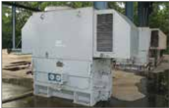
EM3554 1400 KW Toshiba 6 Pole Electric Motor: 985 RPM - CACA
